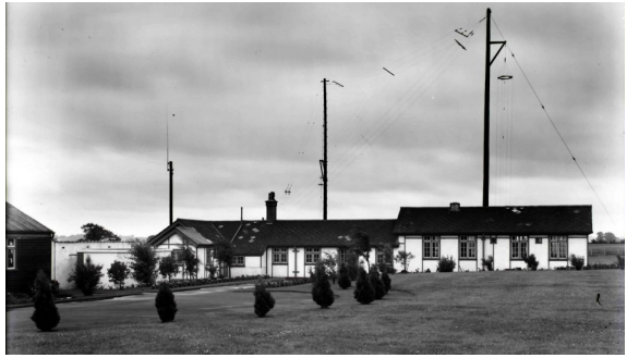
Banbury Radio Station Block A building, north west facing side, 21 August 1954. The original early 1920s building appears to have gained an additional porch compared to the original plan (Reproduced with permission from BT Archives)
