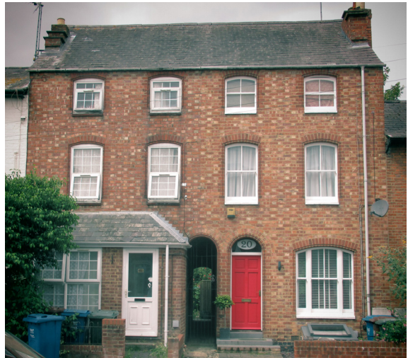
19-20 Centre Street, Grimsbury that were under construction in 1901 half a century after the plots in the street had been laid out by the Freehold Land Society
