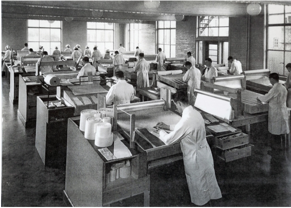
Cutting room on first floor of Wallis, Gilbert and Partners extension (Sheila Evans)
