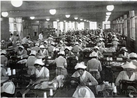
Work room on first floor of new wing (Sheila Evans)
